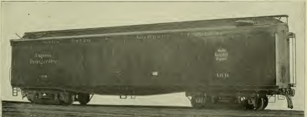
Wells, Fargo & Company Refrigerator Car for Express Service.
